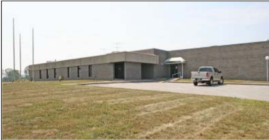
The Therm-O-Disc Building is pictured above.
