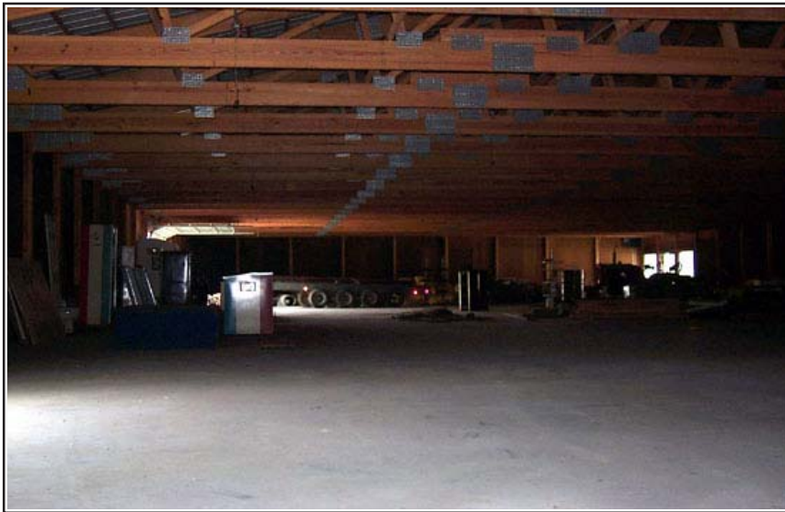
Interior view of Don Bailey Facility in Magoffin County
