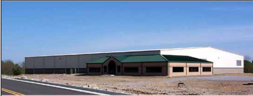
Exterior photo of the Honey Branch Spec Building in Martin County
