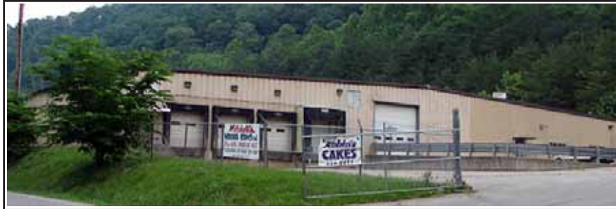
Shown above is the exterior view of the Hobbs Warehouse in Pike County.
