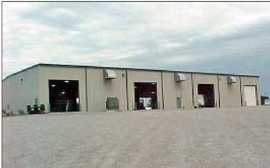
The back of the Lippert Building is pictured above.
