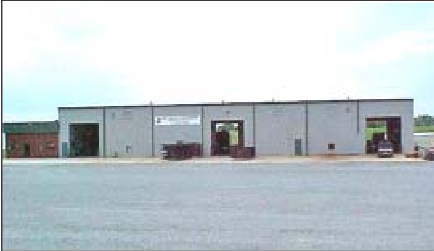
The front of the Lippert Building is pictured above.
