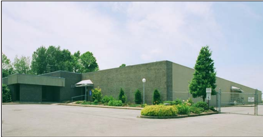
The Therm-O-Disc Building is pictured above.
