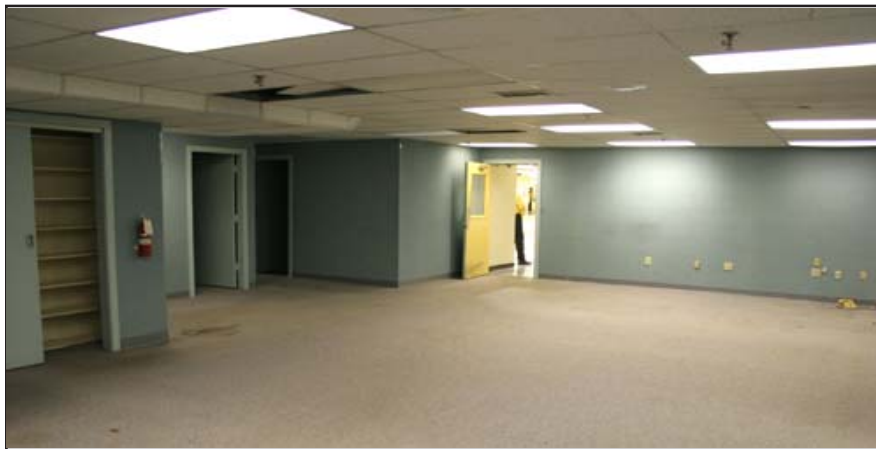
An interior view of the building is shown above.
