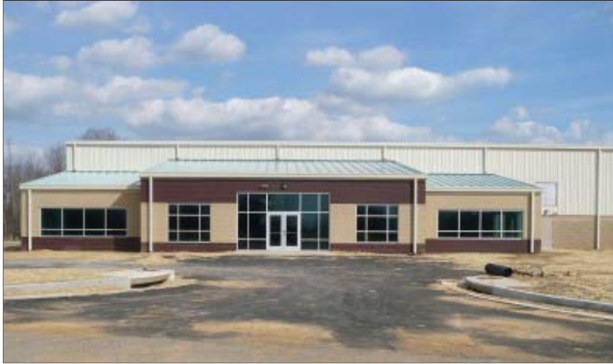
The exterior view of the Russell County Speculative building is pictured above.
