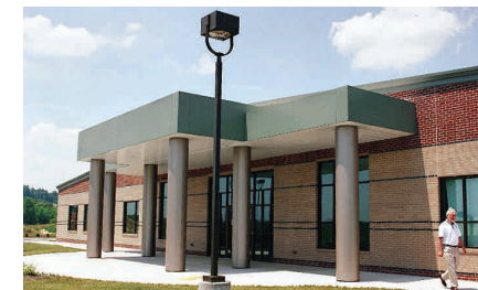
SAIC began operations at the Valley Oak Technology Complex in 2005.
